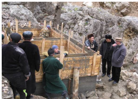
Construction of drinking water system in Yori, Penjikent | GTZ
